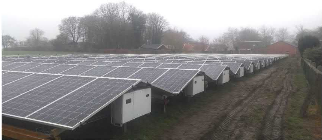
Photo 1-4: Solar panels with east-west facing configuration (image reproduced courtesy of Huawei)
