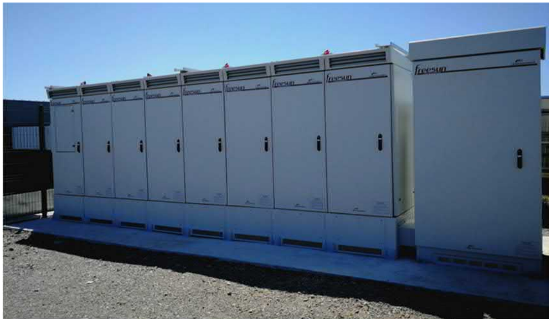
Photo 1-9: Typical outdoor centralised inverter (as per Supporting Infrastructure Option A)
