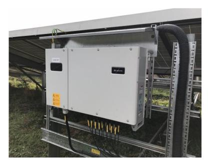
Plate 2-6 Typical string inverter (image reproduced courtesy of Huawei)
